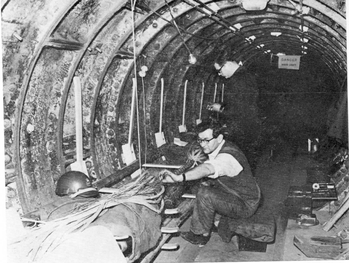
LTR technicians joining cables in one of the seven-ft diameter tunnels beneath Oxford Circus. Each tunnel is about 300 yards long. All tunnel shafts and manholes are electrically lit and ventilated.
