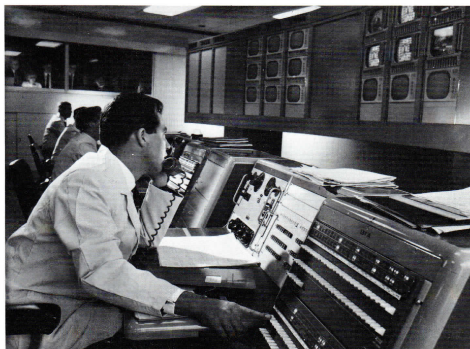
Testing operations in the Television Network Switching Centre. All circuits are terminated in this control room. Engineers are seated at the Test Consoles, where suitable test gear can be connected to any circuit. The switch key being operated in the foreground connects the circuit under test to one of the picture monitors seen in the suite beyond, enabling the engineer to assess the performance of the circuit.
