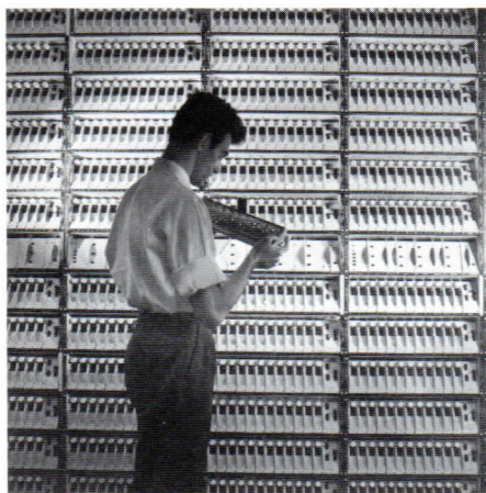
Inspection of a channel panel. One of these plug-in units is needed for each of the thousands of telephone trunk circuits brought into the Post Office Tower.
