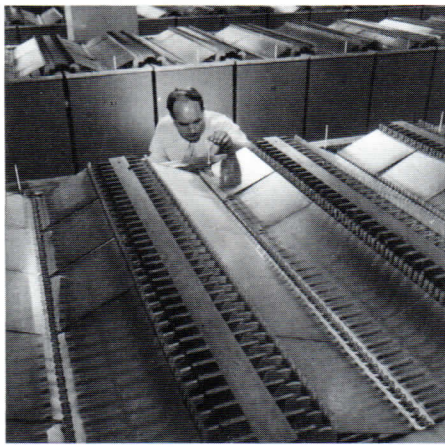
Inspecting the batteries: a maintenance man reads a hydrometer, an instrument for testing the specific gravity of the acid, in one of the very large cells. Batteries of these cells form an integral part of the power plant serving the telephone switching equipment.
