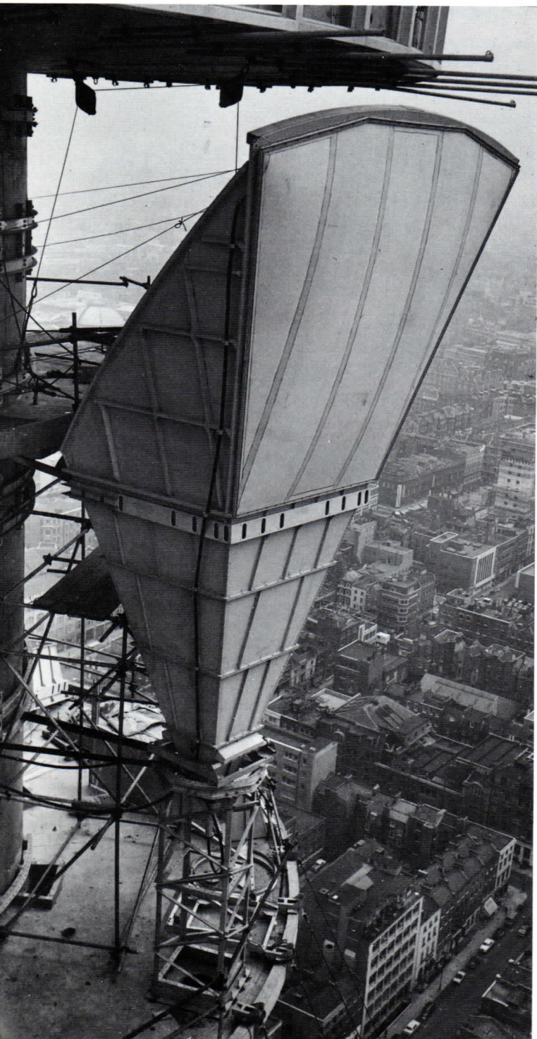
One of the horn aerals being fixed in position.
