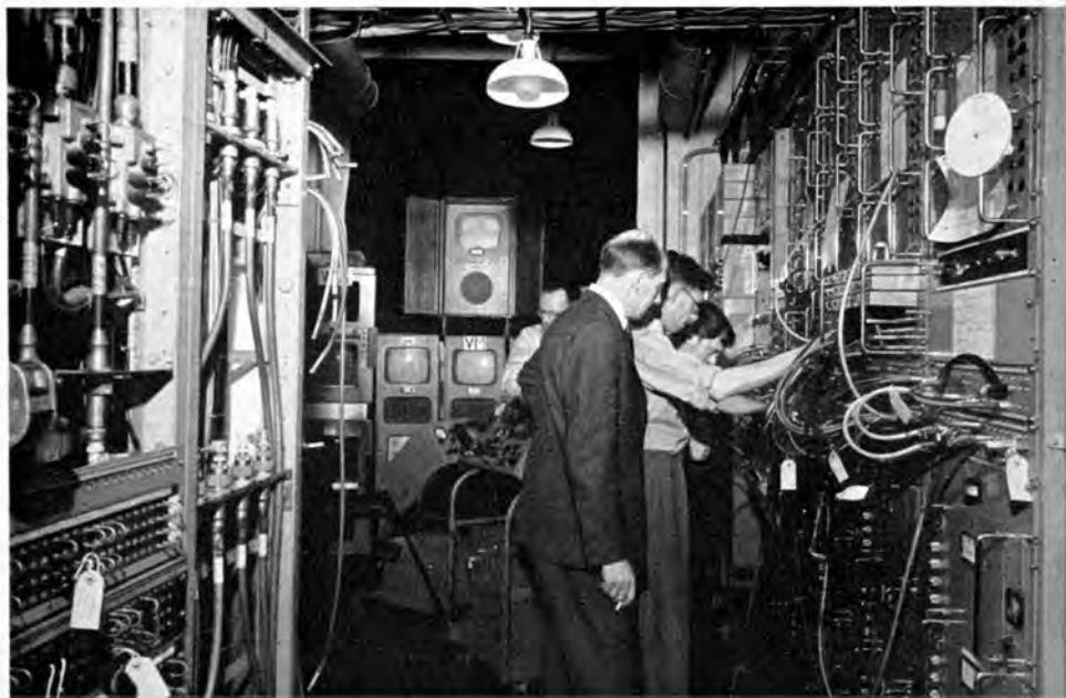
THE TELEVISION SWITCHING CENTRE AT BROADCASTING HOUSE
