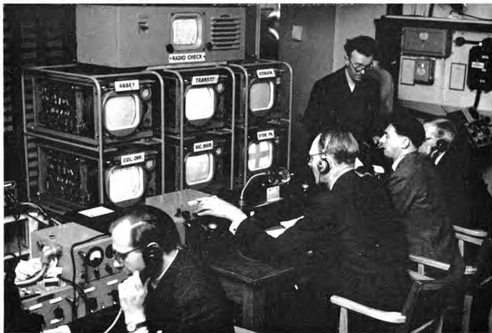
THE TEMPORARY CENTRAL CONTROL ROOM IN BROADCASTING HOUSE
